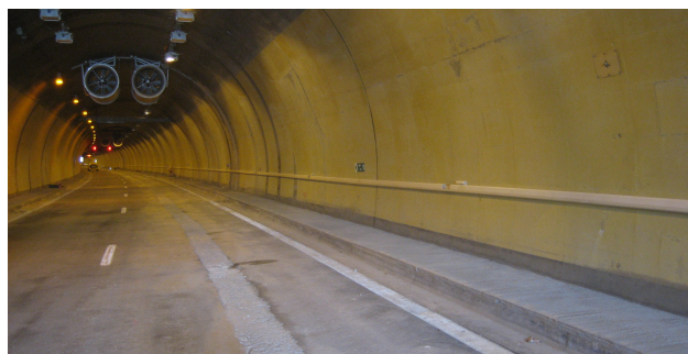
Tunnel A40 — intervention EXTHA
